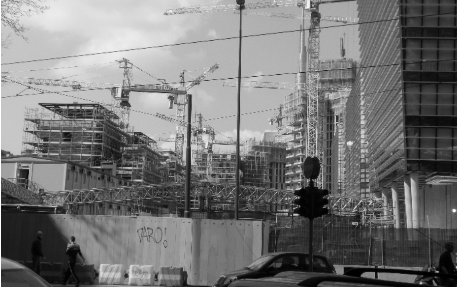
Figure 3: Construction site of one of the new development projects in Milan.
