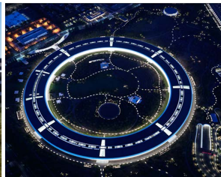
Figure 14. Apple HQ survey pic 4. Source: Pinterest
