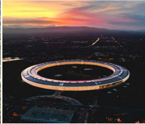
Figure 12. Apple HQ survey pic 2. Source: Pinterest
