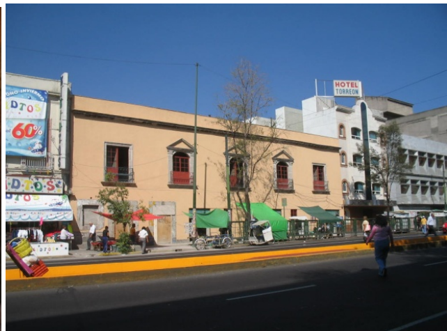
Fig. 16. Fachada rehabilitada Rehabilitated facade.
