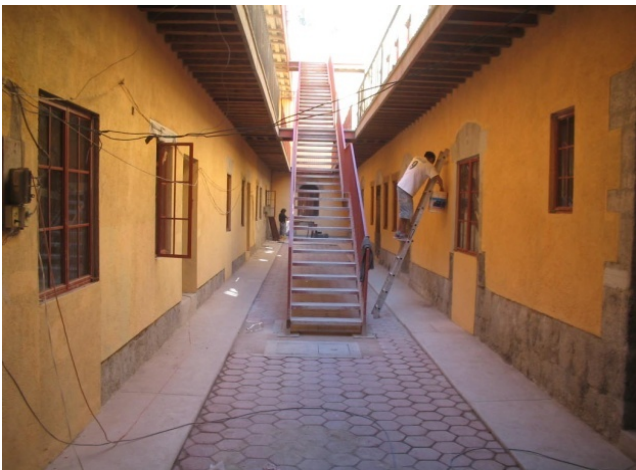
Fig. 15. Aplanados terminados. Renderings finished before painting.
