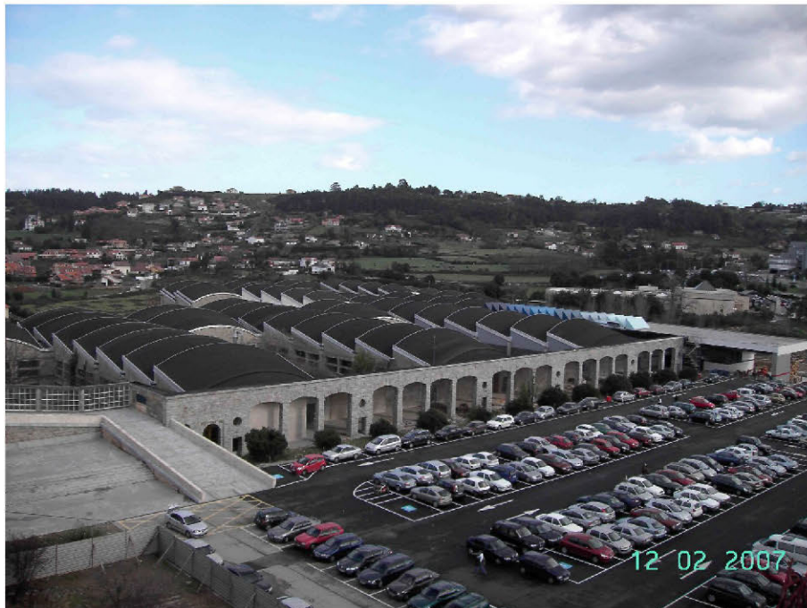
Figura 2. Pórtico en la fachada principal de los talleres. Figure 2. Portico on the main facade of the workshops.
