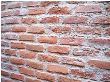
fig. 7 reintegración superficial con mortero y pintura ( re-integration of missing parts by means of mortar and paint )
