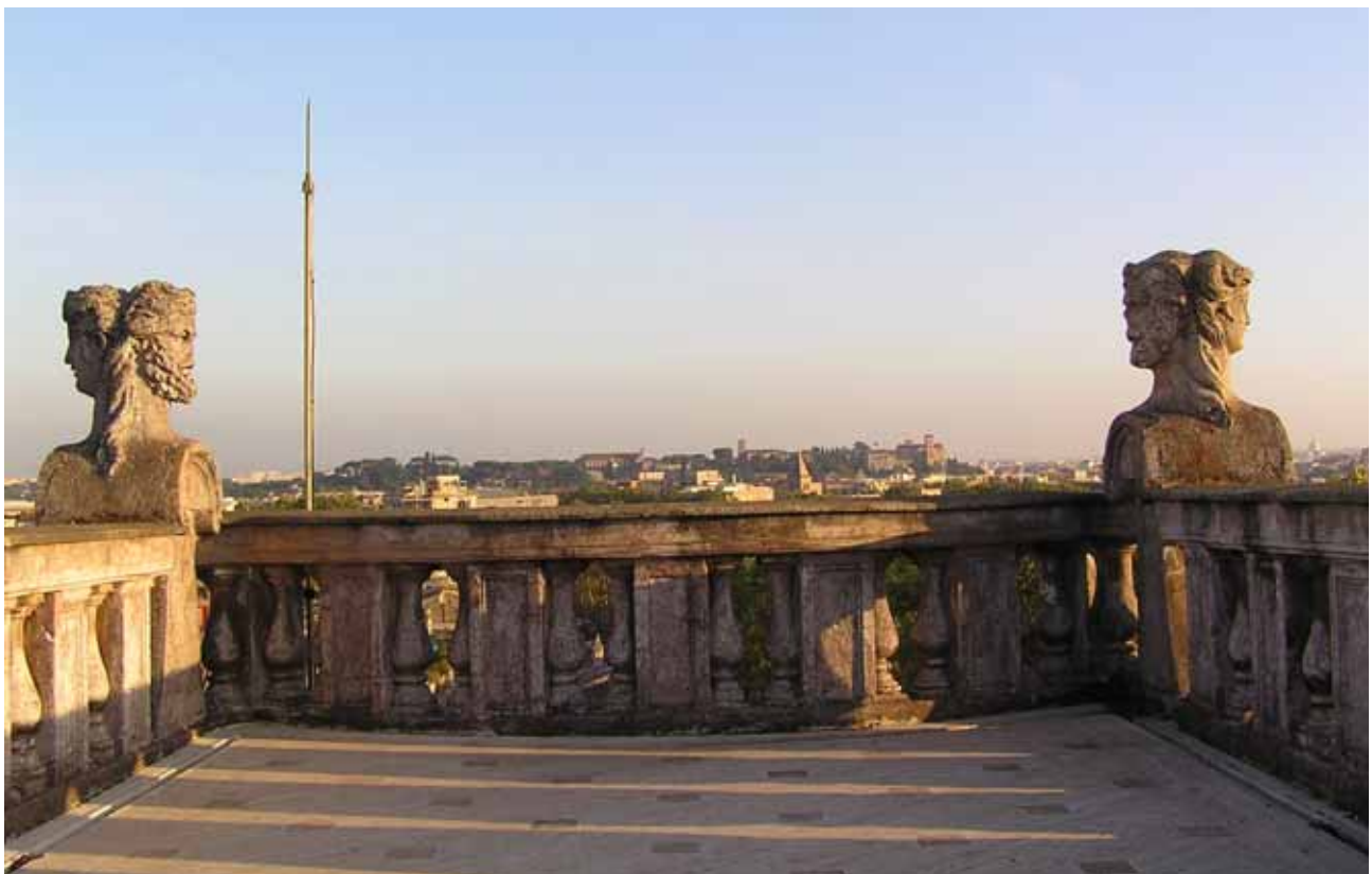
Fig 12. Extremo concavo del belvedere. Concave extreme of terrace.
