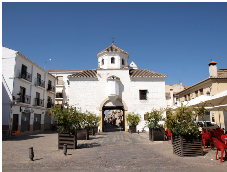
Figure 4. Left page. Santa Fe, Gate of Granada. Outside view. Built in the 17th century after the collapse of a previous structure. It was designed as a gated chapel, with a domed main altar placed over the door. Author.
