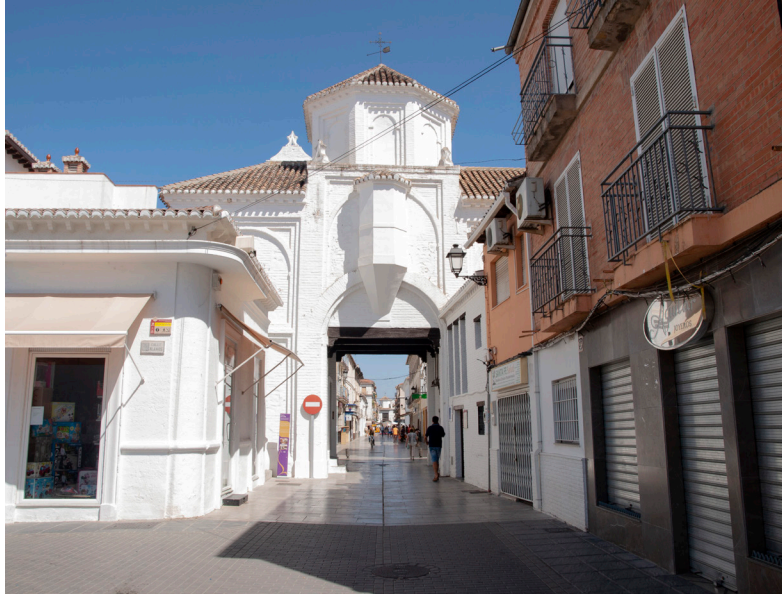
Figure 5. Santa Fe, Gate of Seville. Outside view. Author.
