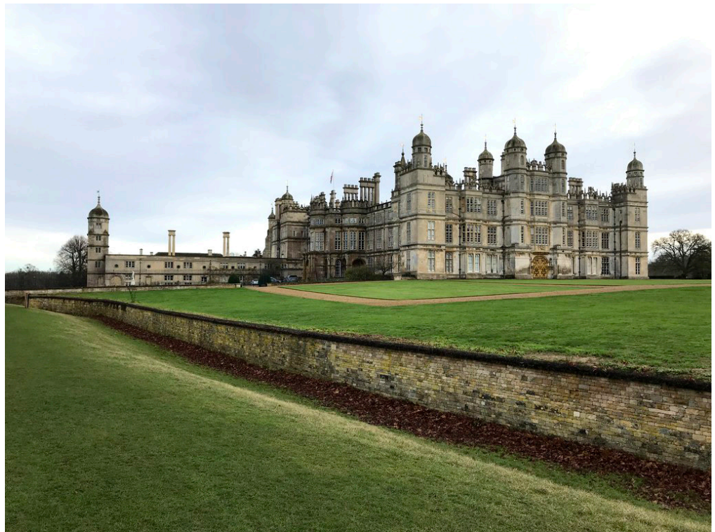
Figura 21. Burghley House, Stamford. Ha-ha realizado por Capability Brown, s.XVIII. Copyright Richard Humphrey and licensed for reuse under Creative Commons Licence.
