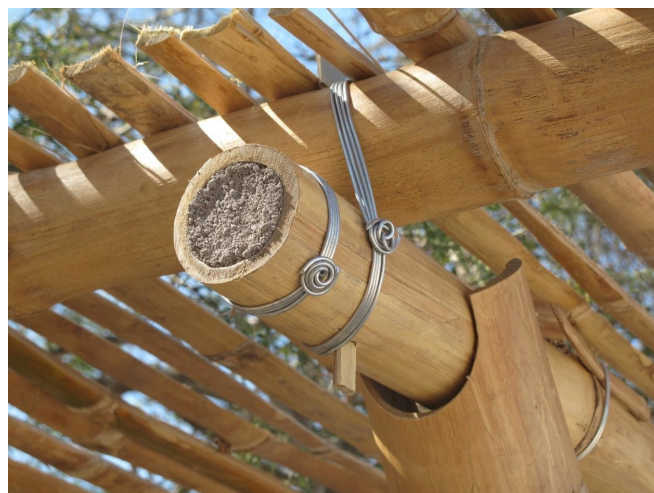
Fig. 27. Detalle constructivo 1 Tomado de Playa Man - the Scarcity and Creativity Studio [8]
