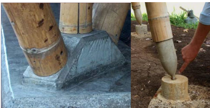
Fig. 24. Detalle constructivos Tomado de Playa Man - the Scarcity and Creativity Studio [8]
