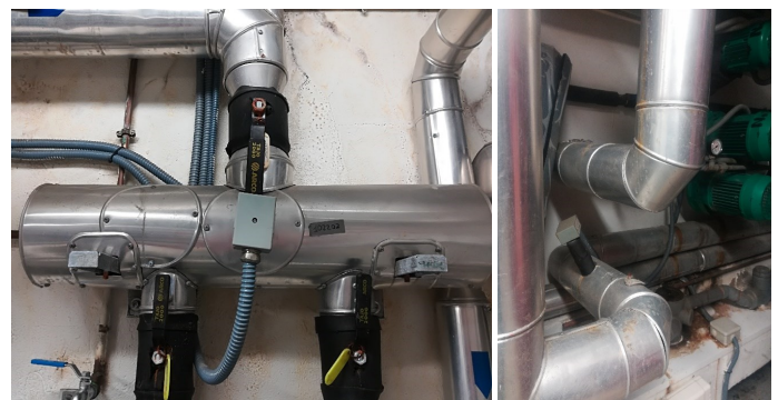
Figure 10: MAMAC SYSTEMS - TE-703-B-17-B-2 - Pipe Temperature Sensors. Apolonio Morales 29, Madrid, Control System. Source: Self-elaboration.
