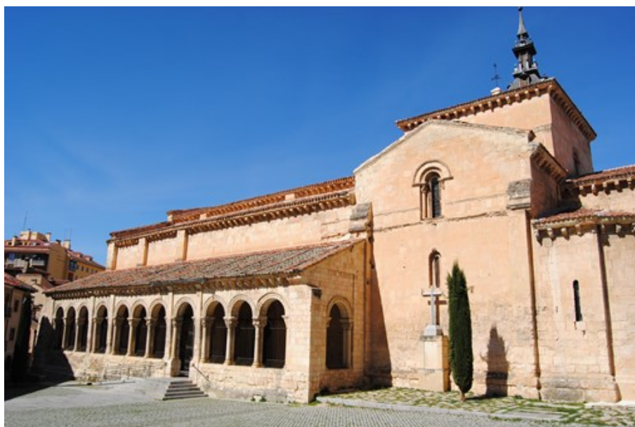
Figure 1. South façade and atrium of San Millán de Segovia.
