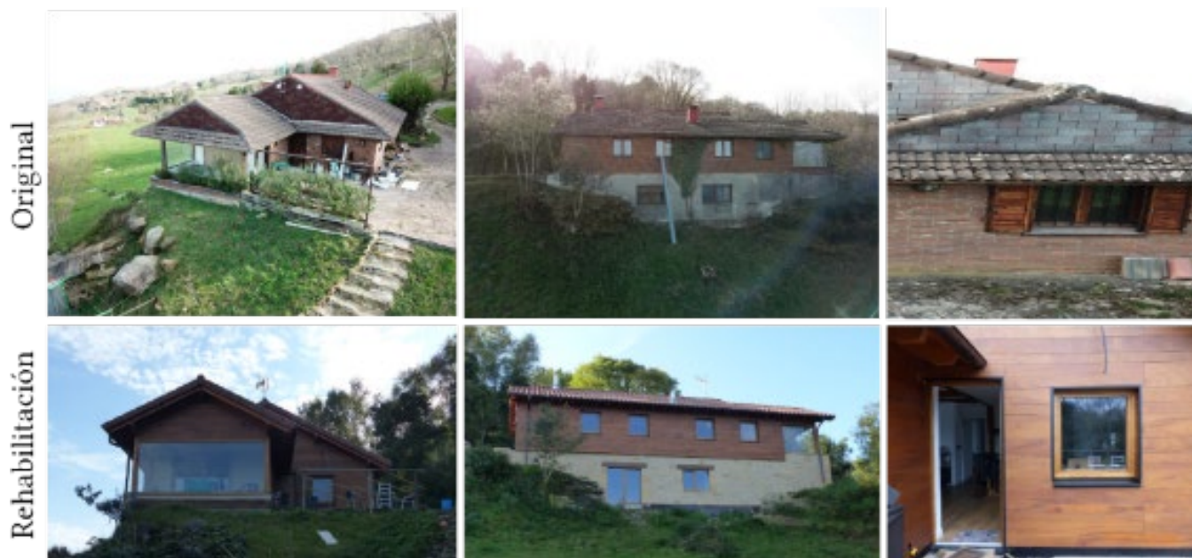
Fig. 2. Original and rehabilitated state of the case study (Source: Own authorship)..
