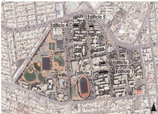
Fig. 2. Selection of CAPFCE Buildings at the Hermosillo Campus of the University of Sonora. Made with image from Google Earth (Google Earth Pro, 2024).
