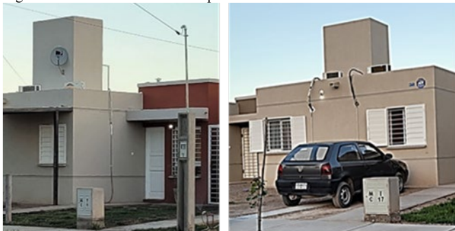
Fig. 2. VSE-IPV West Facades with or without Covered Carports and Active AC Equipment on Roofs
