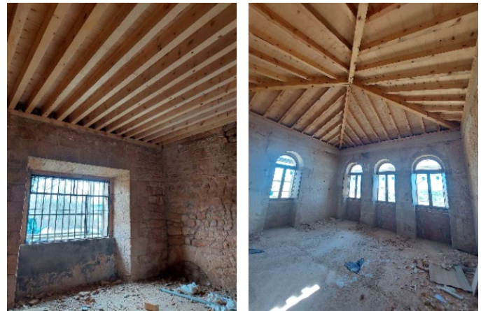
Fig. 17: Rehabilitation of the structure. (Source: Paula Montoya Saiz)
