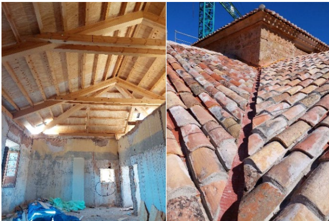
Fig. 16: Rehabilitation of the roofs. (Source: Paula Montoya Saiz)
