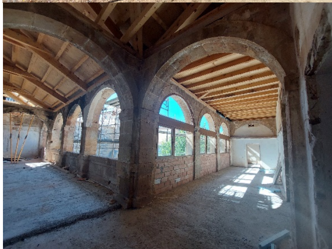
Fig. 18. Rehabilitation of walls. (Source: Paula Montoya Saiz)
