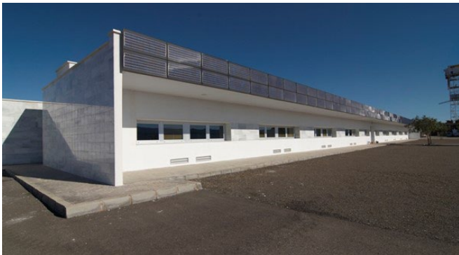
Fig. 2. South main façade of the PSA office building. The studied office room is in the southeast corner, marked with a yellow circle.
