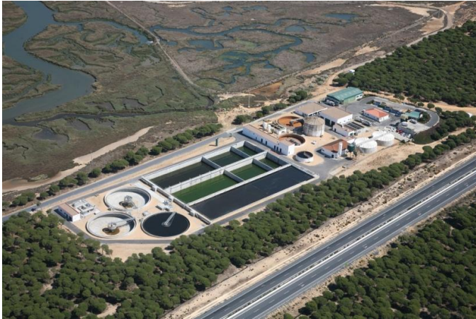
Fig. 7. Odiel Marshes WWTP in 2012 (Source: author).
