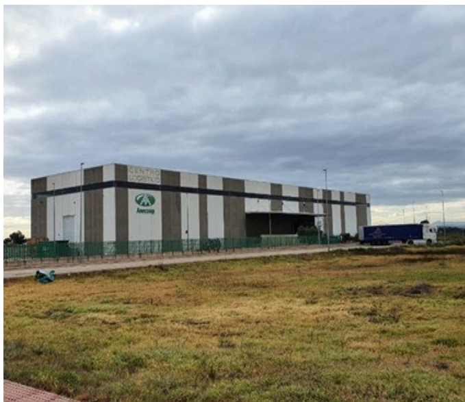
Fig. 4.. Anecoop Logistics Centre S.Coop. (Own elaboration)
