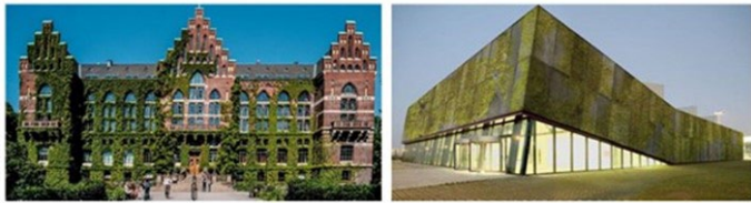
Fig. 11 Unsupported vegetal façade (Lund University, 2022), Hormigón vegetal (Univ. Polit. de Cataluña, 2017)
