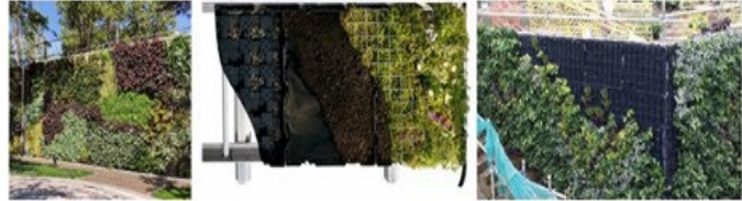
Fig. 13 Bonded support (Singular Green, 2022), pre-cultivated box (Vivers Ter, 2022) and modular block (Scotscape, 2022)
