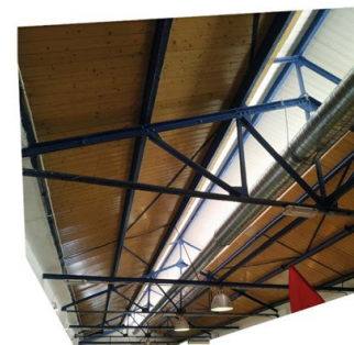
Fig. 21. Structure of the side deck aisle and its available load-bearing capacity. Source: Own elaboration
