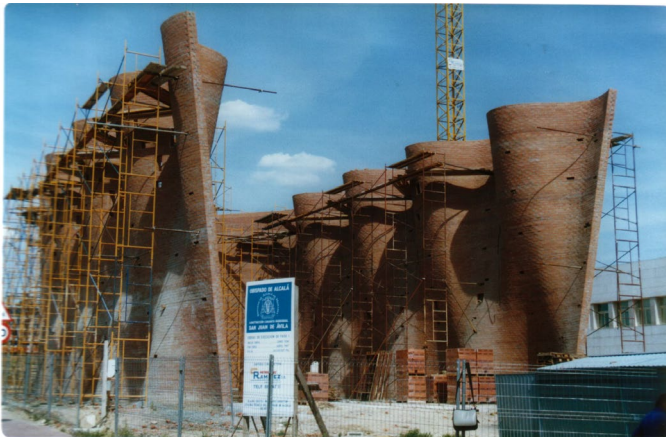
Fig. 8. San Juan de Ávila church construction process. (Lávila, 2018)
