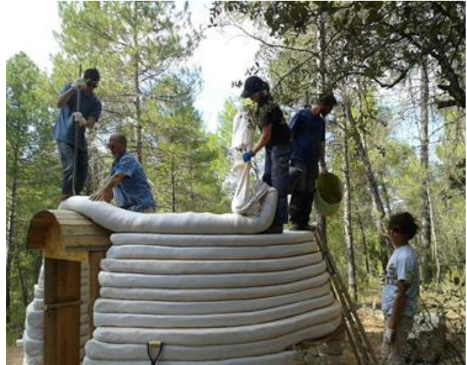
Fig. 12. Stomping the ring.
