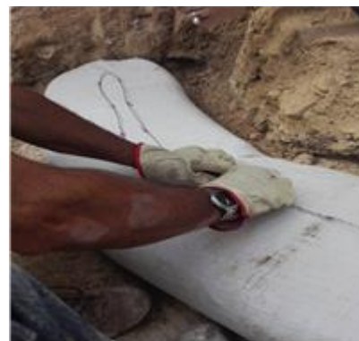
Fig. 13. Stitching barbed wire to the ring.
