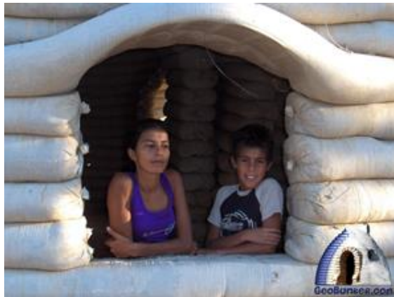
Fig. 17. Window opening after removal of the mold. Notice the self-sustainable arch form of the window according to the steps described above.
