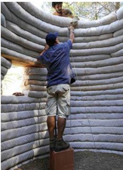
Fig. 10. Measuring correct distance of the ring edge with the central compass.
