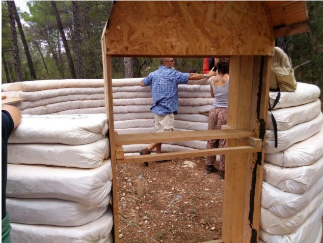
Fig. 14. Mold / Frame for the main door.
