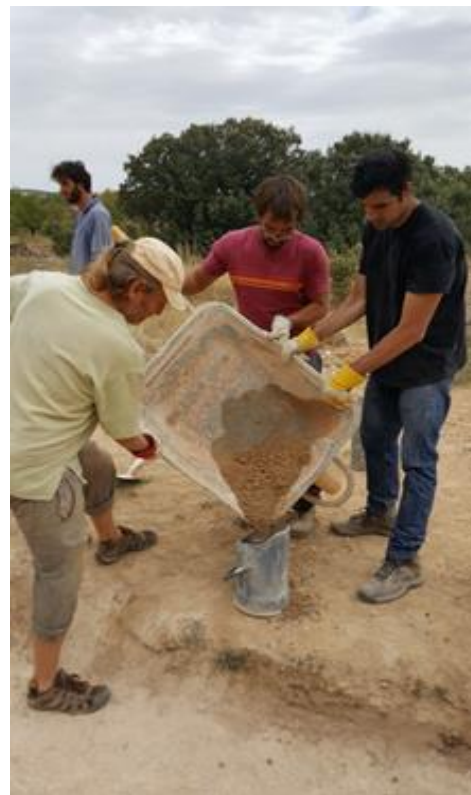
Fig. 8. Delivering mixture to the dome area.
