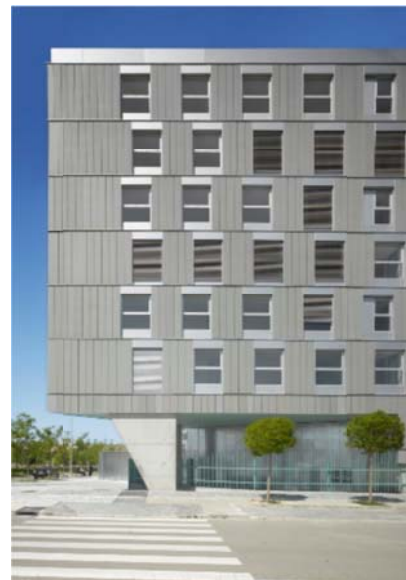
Fig. 2. General view of the building.
