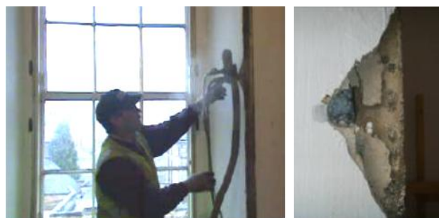
Fig. 5. Pressurized expanded polystyrene bead insulation in walls.
