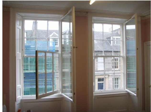
Fig. 7. Secondary aluminium windows behind existing sash & case timber windows.
