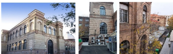
Fig. 19: Details of the back part of the building of the 'Palace of Industry and Fine Arts' at present time (Source: Photographs by G. Pinto).
