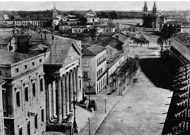
Fig. 9: Church and Convent of the Holy Spirit, demolished in 1842, and the Palacio de las Cortes in 1853. (Source: Above- Wikimedia Commons; Below - Pinterest. Public domain).
