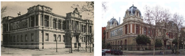
Fig. 12: Building of the School of Mining Engineering at the end of the 19th century and presently (Source: Left - Wikimedia Commons. Public domain; Right - https://short.upm.es/ti0n0 CC BY-SA 3.0).
