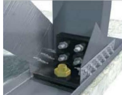
Fig 9: Connections using screws (source:16)
