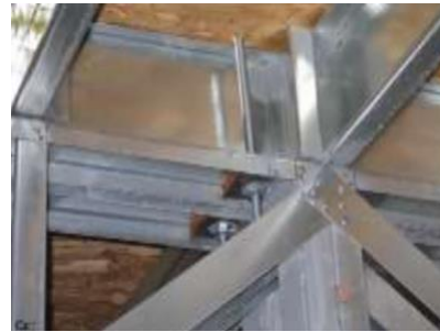
Fig 10: Connections using screws (source:16)
