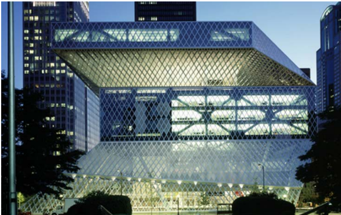
Fig. 2. Exterior Image, Seattle Library (Source: OMA)
