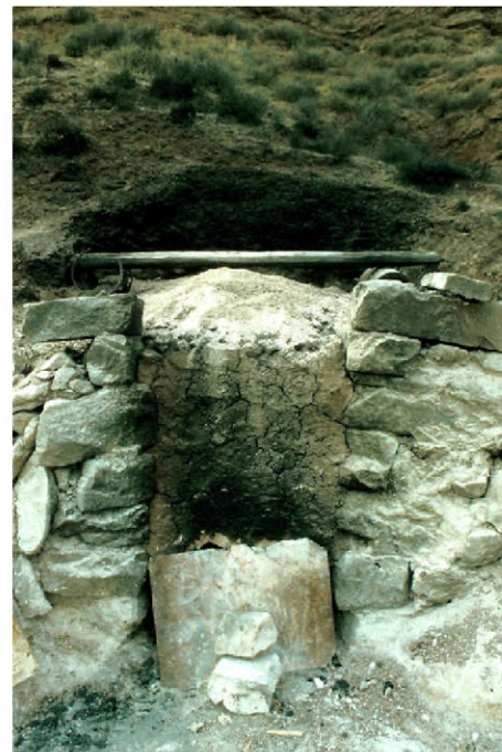
Figura 15. Horno de Albarracín (Teruel), recubierto de barro y apagado a la espera de ser desmontado. Figure 15. Kiln in Albarracín (Teruel), covered with mud and put out, waiting to be dismantled.
