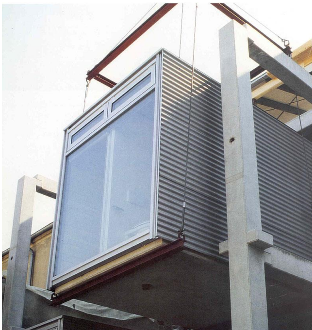
Fig. 27. Retrofit offices at Hamburg, 1999.
