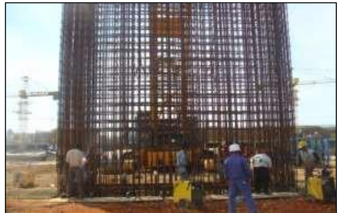
Fig. 2. The welding of strips of reinforcement.
