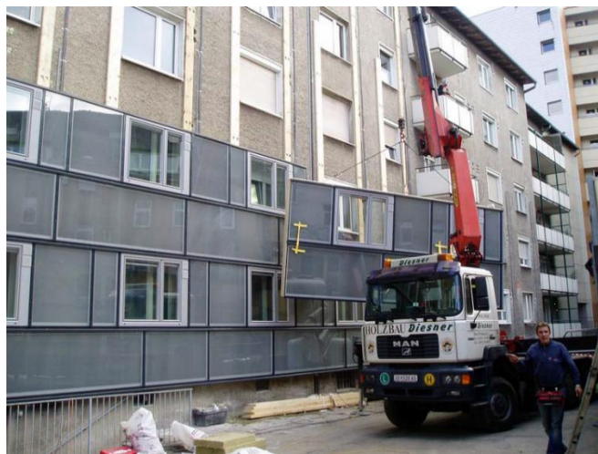
Fig. 3. Installation of large panels on Makartstrasse building.
