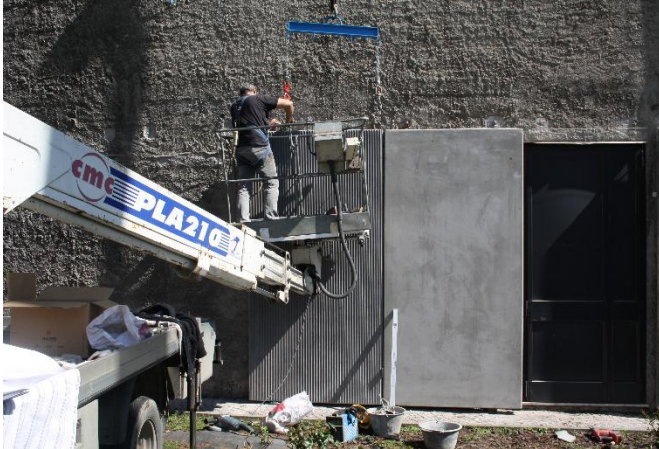
Fig. 4. Installation of EASEE panels on case-study building.
